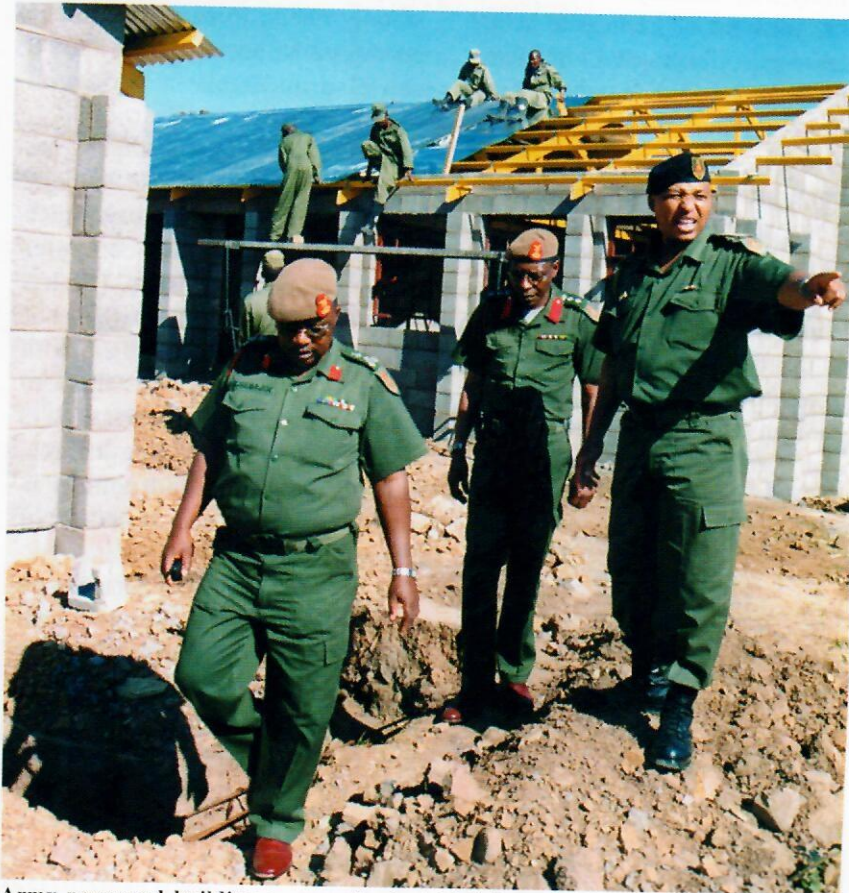
Army personnel building a new school at Maliele
